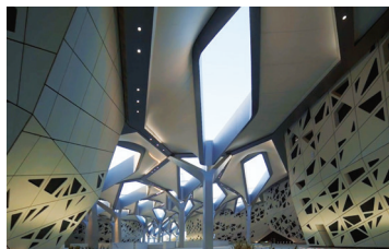
3D Shaped, Aluminium Composite Panel Cladding
