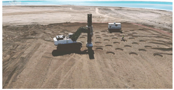
Compaction work in progress at the Red Sea site.
