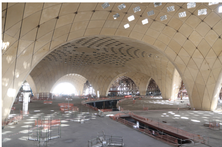
From concept (above) to construction ... all the 36,964 shell cassettes required for the interior roof of the terminal have been installed.
