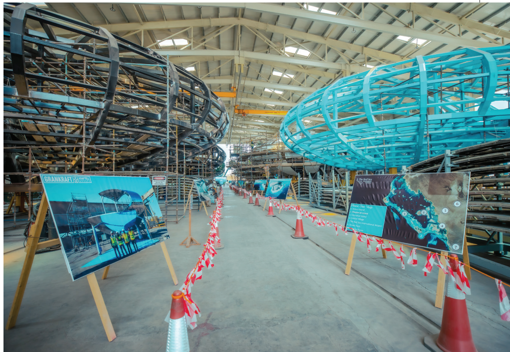
Hidden within the orbs is an extensive steel superstructure.
