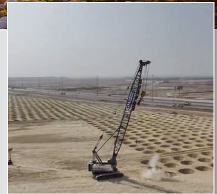
The Mukaab ... centrepiece of the New Murabba development. BELOW: Dynamic compaction work under way on site.
