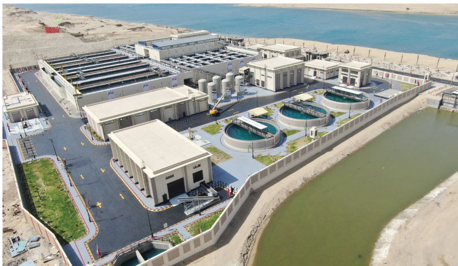
Egypt's Al Mahsamma plant ... the largest of its kind in the world.
