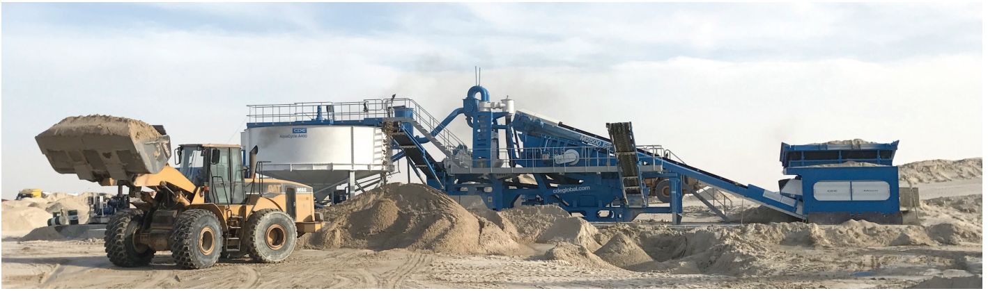
CDE has 75 wet processing plants successfully utilising its water management and recycling technology in the Mena region.
