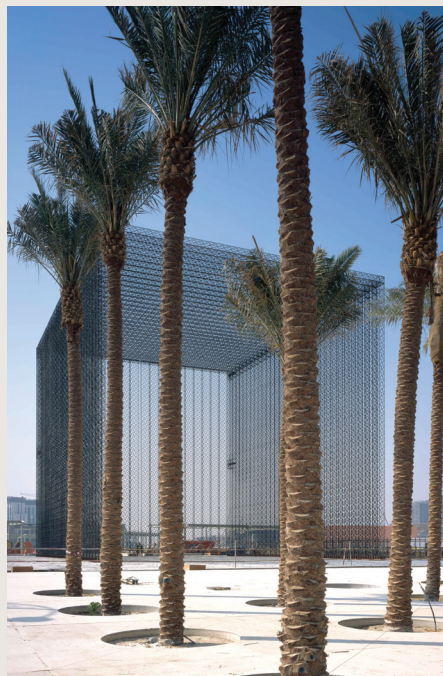
The 21-m-high and 30-m-long portals ... woven from strands of ultra-lightweight carbon-fibre composite.
