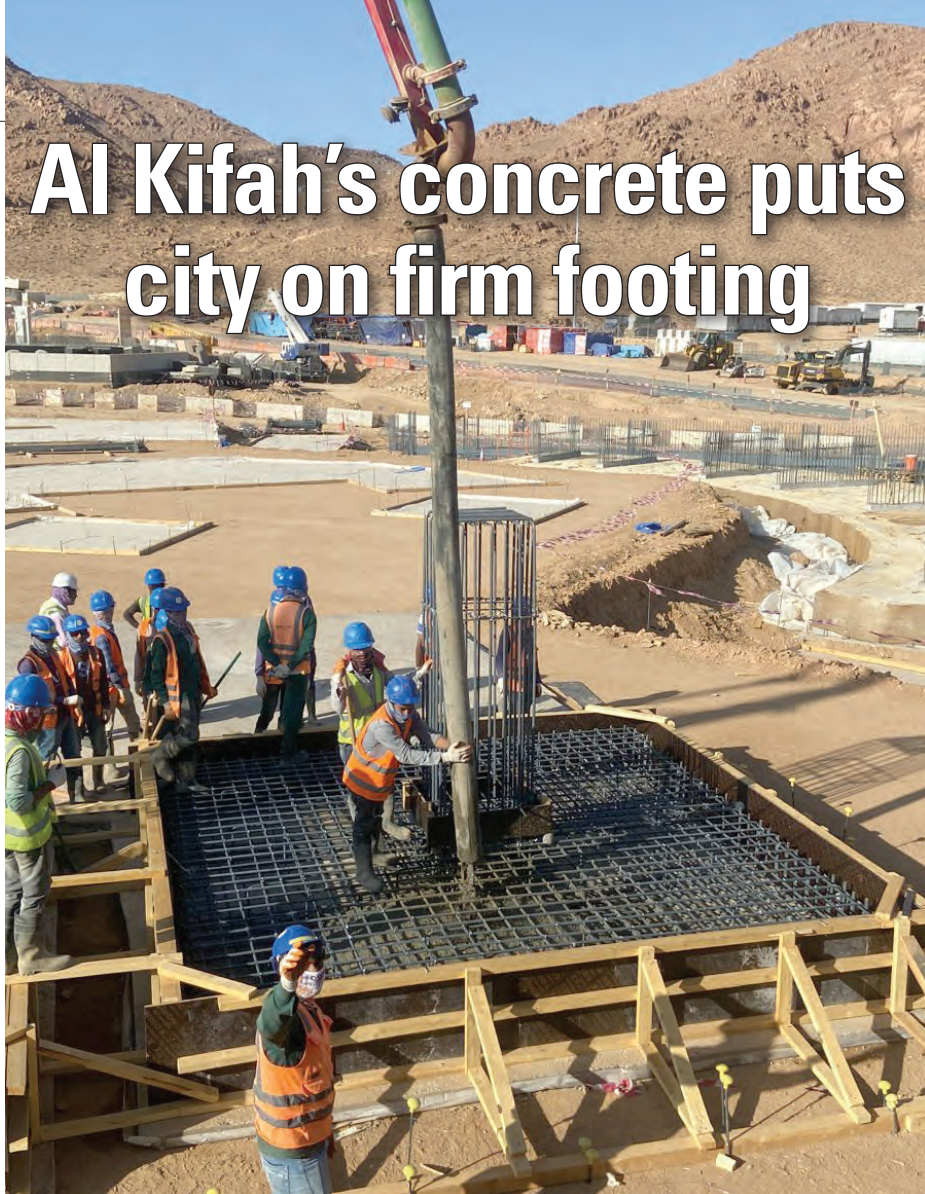
The first concrete pour for the project was carried out on March 3 this year.
