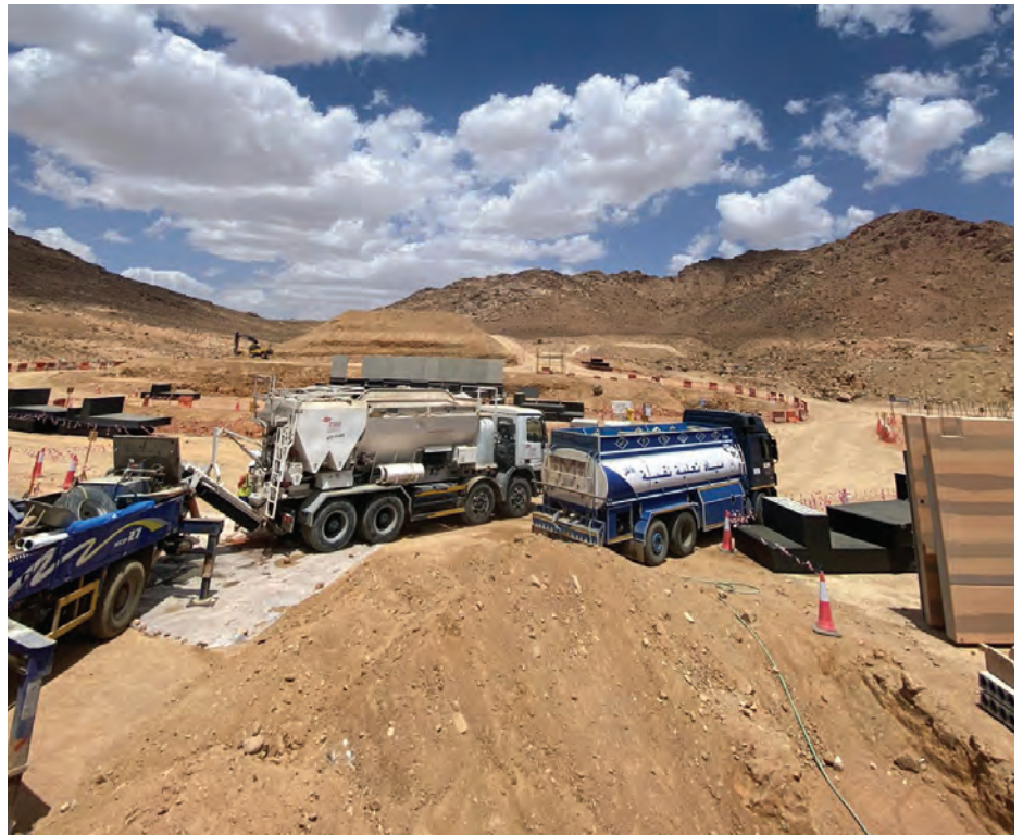
KRB has deployed Volucon Volumetric Mobile Batch Plants to produce high-quality concrete that conforms to international standards.
