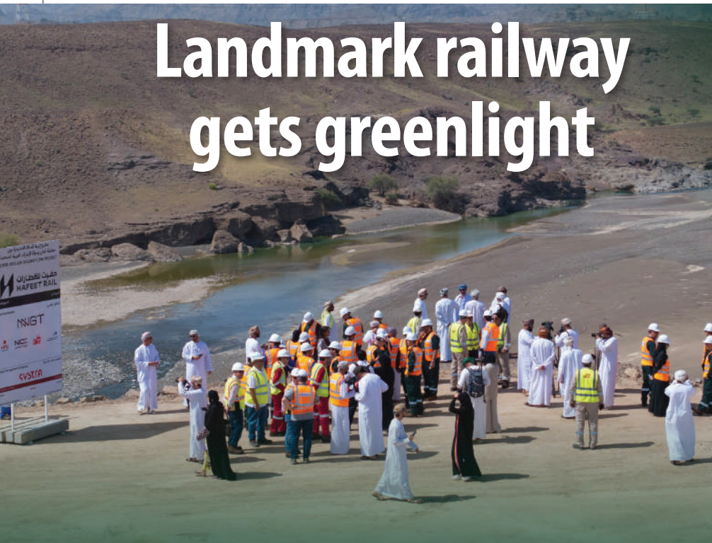
A construction site of the railway was visited by senior officials of stakeholders.
