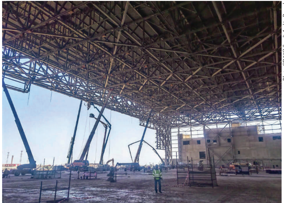
Installation of the steel structure of a heavy maintenance hangar of King Abdulaziz International Airport.
