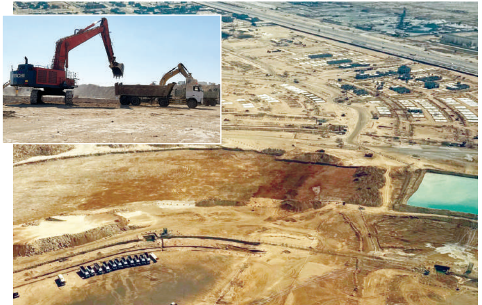
Excavation work is currently under way on Marafy's 11-km canal.
