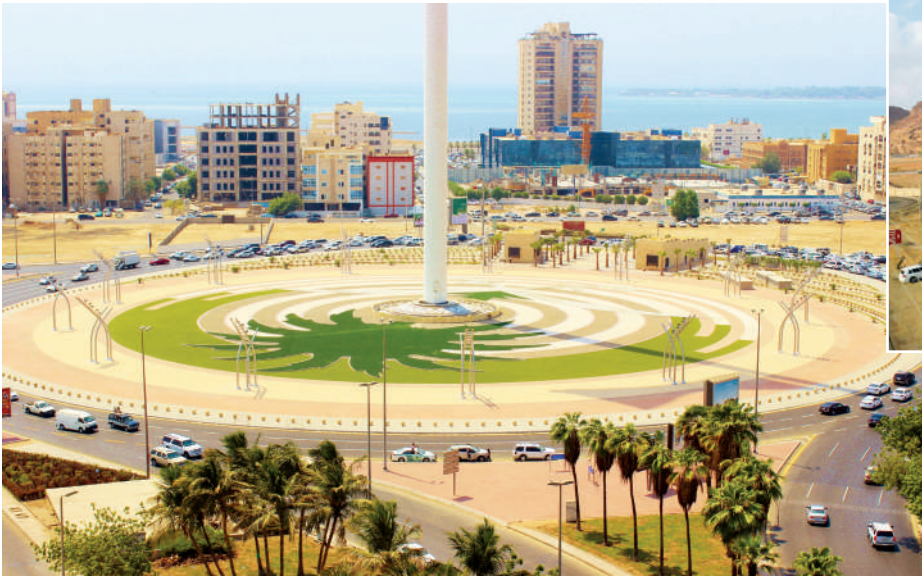
Mattex has supplied to significant projects across Saudi Arabia.
