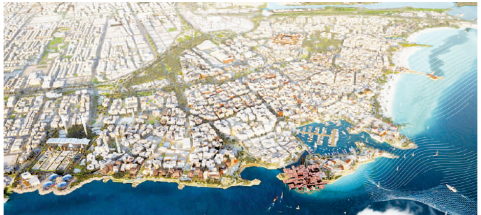
Jeddah Central project spans a 5.7-million-sq-m plot of land overlooking the Red Sea.
