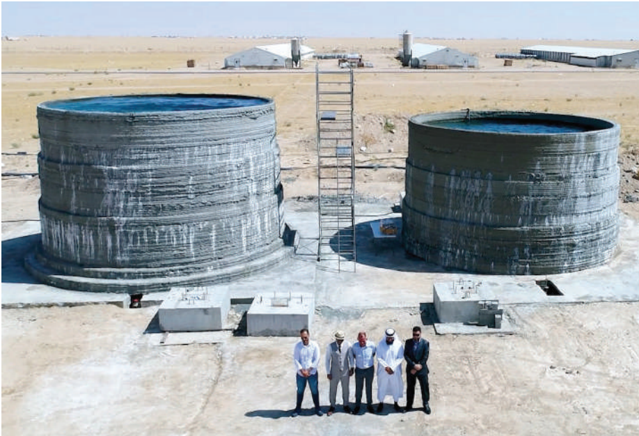
Representatives of Abyan, Cobod, and Kuwait United Poultry Company are seen in front of the world's first on-site 3D printed large water tanks.
